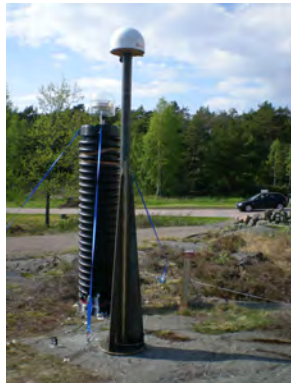
(a) Mast construction
