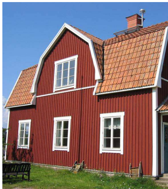
Figure 1.3: Söderboda is a SWEPOS station with a roof-mounted GNSS antenna mainly established for network RTK purposes belonging to class B.
